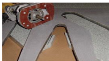
(8) Rout out cracked build up
